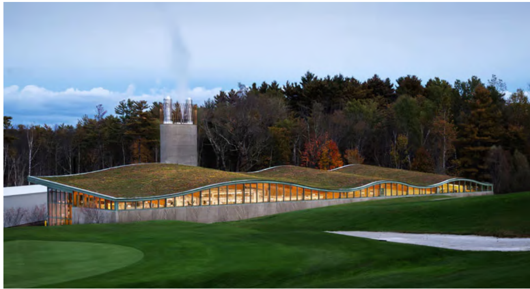
Hotchkiss School Biomass Treatment Facility
