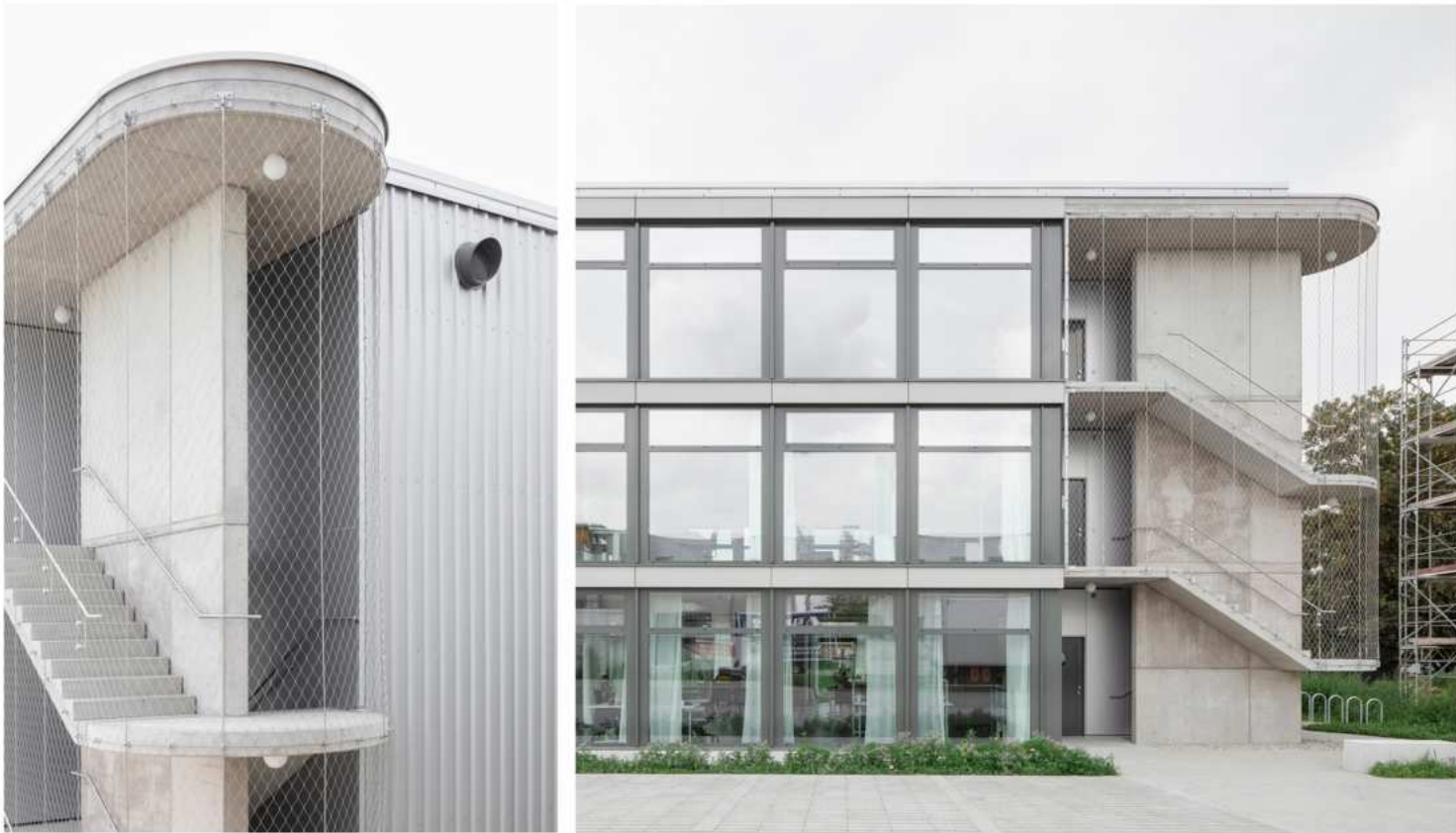
TINA – Flexible Office and Residential Building, Breisach, Germany / STUDIO SOZIA
