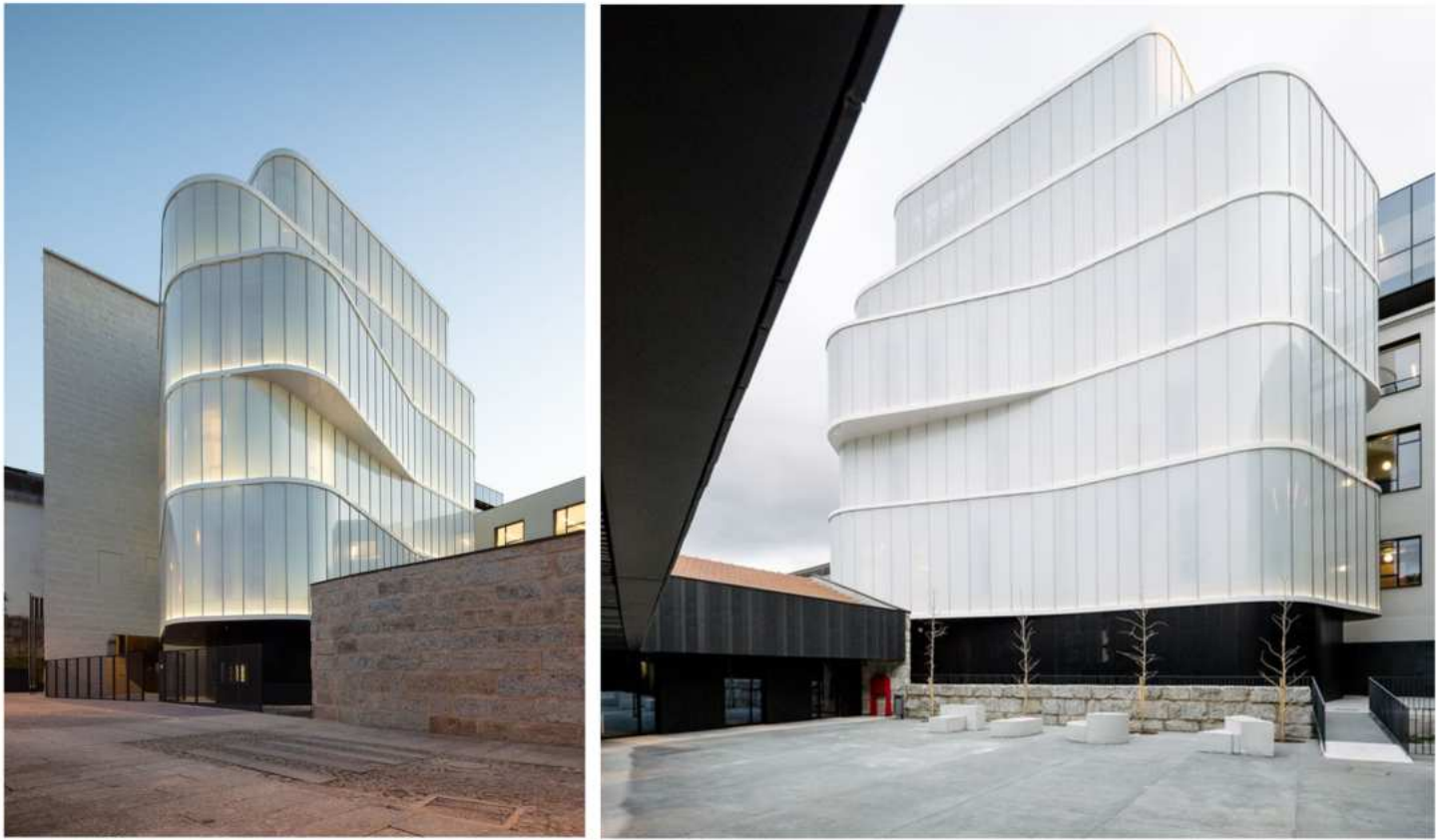
Rehabilitation of the old Jordão Theater and Garage Avenida / Pitagoras Group
