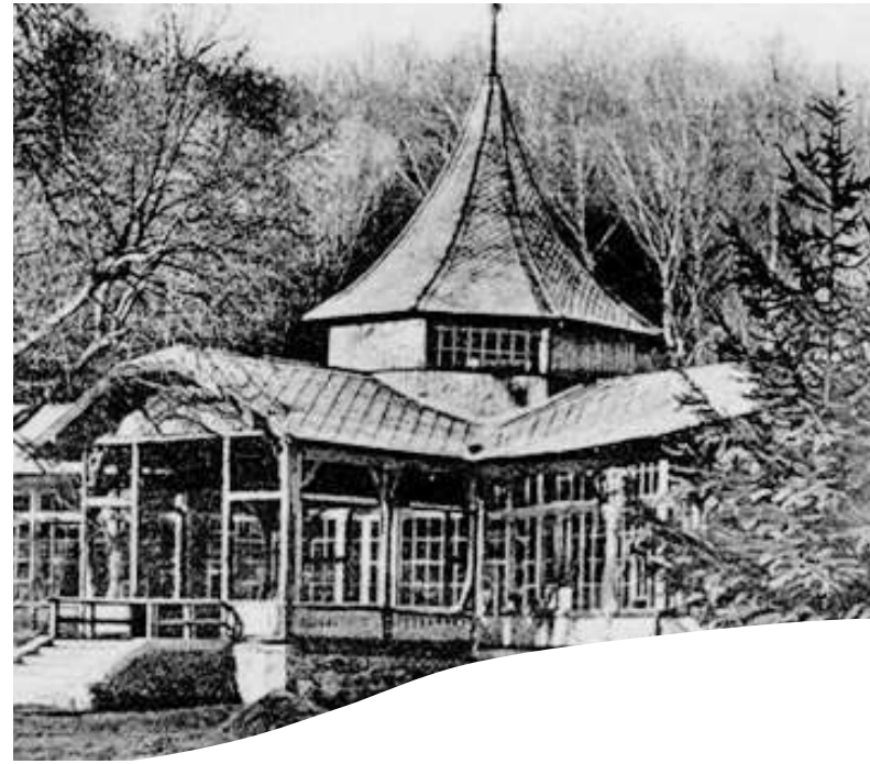
Ferdinand's spa with natural iron water
