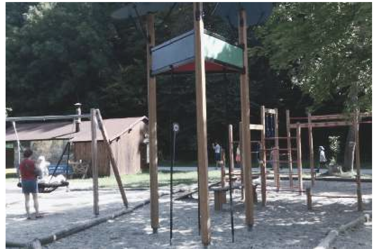
missing shading structure and benches
