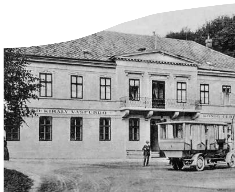
spa rebuilt into a hotel for social events
